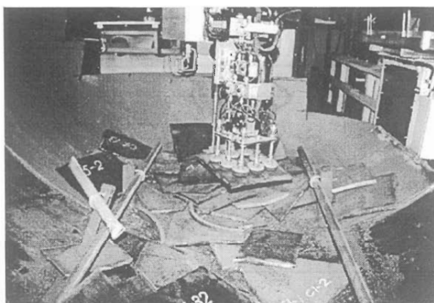
Photo 4 Collection of cut pieces with vacuum pad device
